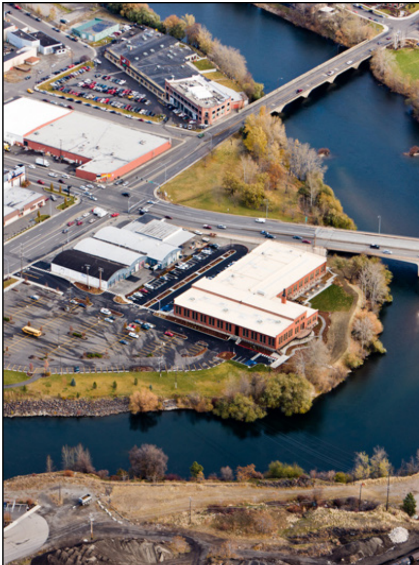
Figure 30: The Spokane and Inland Empire Railroad (SIERR) Building at McKinstry Station after the 2011 renovation, looking to the northeast. Credit: Dean Davis, 2011. Photo courtesy of McKinstry.
