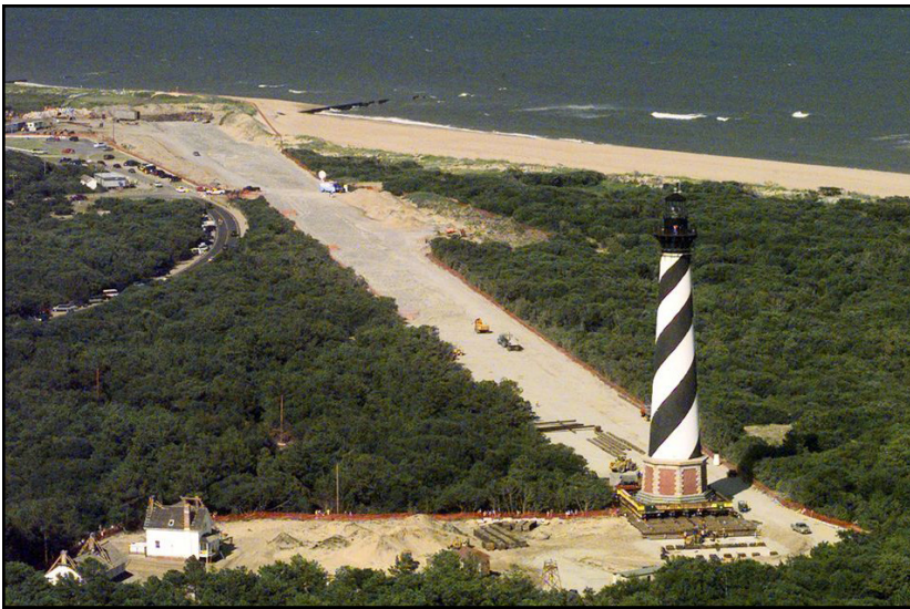
Figure 5: The Cape Hatteras Lighthouse being moved away from the eroding shoreline in a strategic retreat. Credit: www.images.nationalgeographic.com
