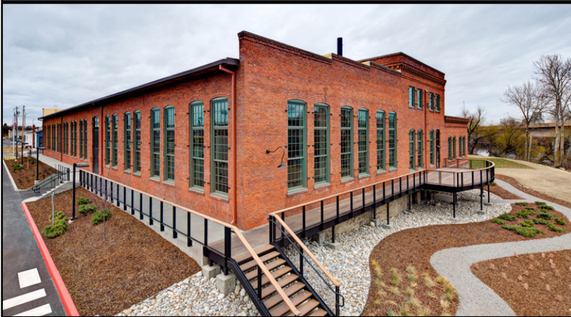
Figure 32: Thousands of cubic yards of contaminated soil were removed from the riverfront side of the site at the right of the photo. Credit: Dean Davis, 2011. Photo courtesy of McKinstry.
