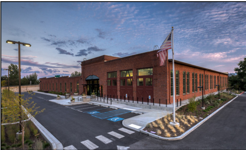
Figure 31: The windows and doors at the SIERR Building were fully reconstructed from existing materials. View looking southeast. Credit: Dean Davis, 2011. Photo courtesy of McKinstry.
