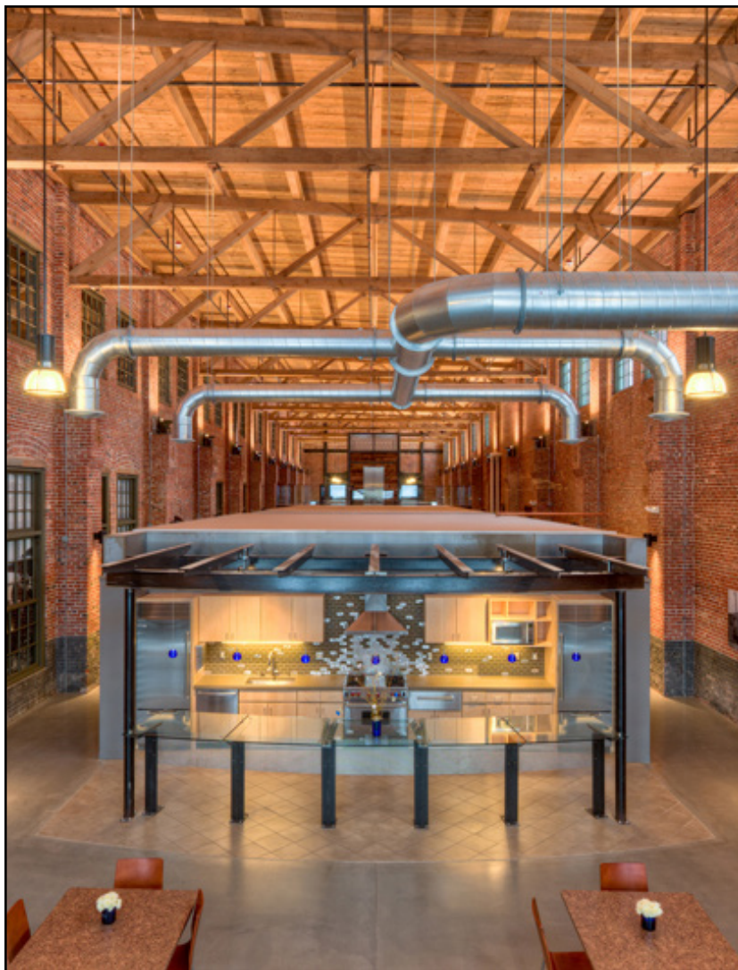
Figure 33: The 2011 rehabilitation made preserved the spacious feeling of the maintenance bays by holding new construction to the center of the space allowing the volume to be clearly understood. Credit: Dean Davis, 2011. Photo courtesy of McKinstry.
