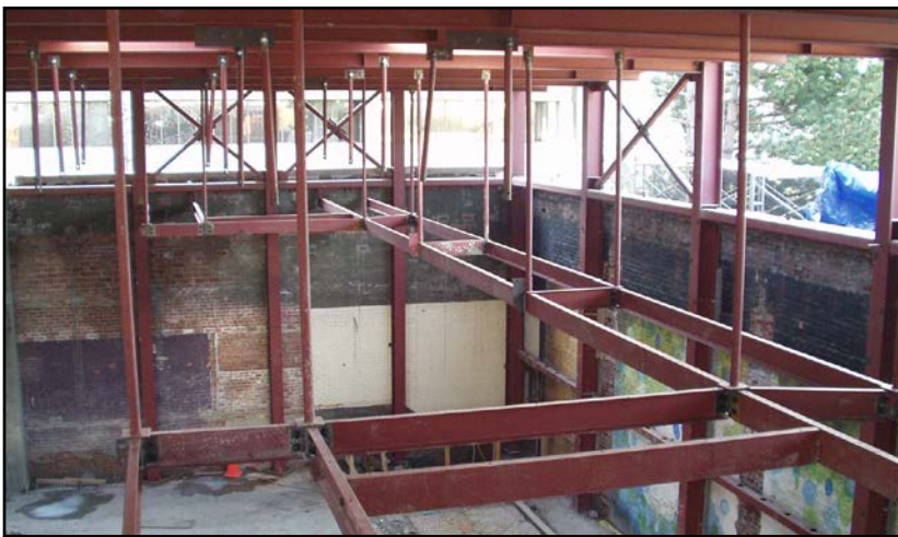
Figure 19: The interior of the stage looking at the catwalks during construction. Credit: Staff photo, UW CPD, 2008.
