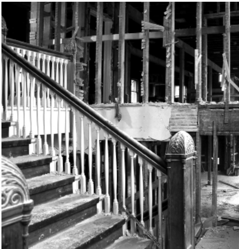
Figure 13: The main staircase in Clark Hall during demolition. Credit: Staff photo courtesy of UW CPD, 2008.
