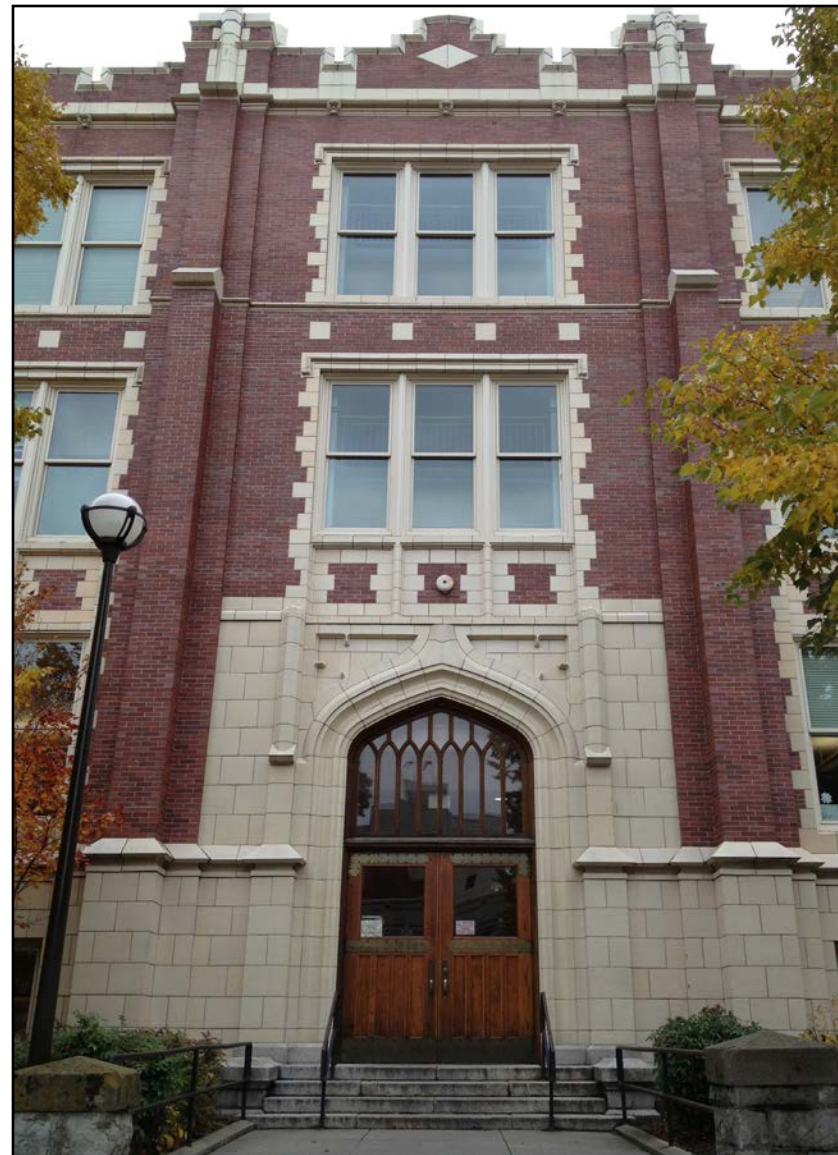
Figure 1: The Lewis & Clark High School in Spokane, WA, was recently renovated. Credit: Brian Rich, 2012.
