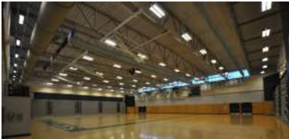
Figure 2: The gym at Skyline High School in Issaquah, WA, is an example of the metal framed roof structure in Gym B and C. Credit: Brian Rich, 2013.
