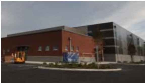
Figure 3: The Gym at Shorewood High school in Shoreline, WA is an example of Gym C construction. The main volume of the gym has CMU exterior walls and metal roof structure. Credit: Brian Rich, 2013.
