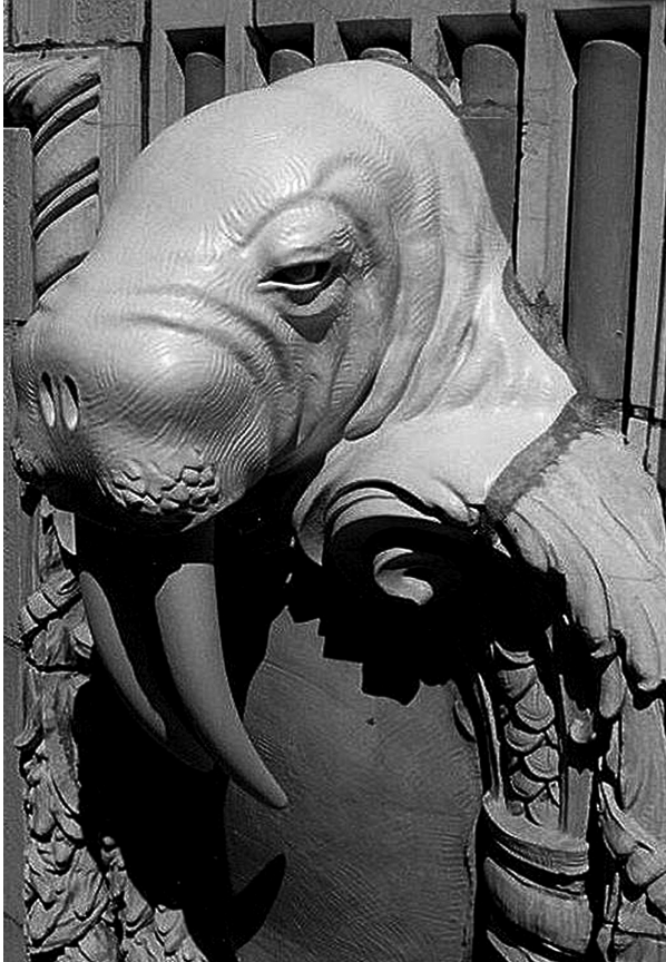
Fig. 8. 1996 replica walrus head. The joints between terra cotta pieces are filled with mortar after the epoxy sets around the threaded rod anchors. (Credit: Wiss, Janney, Elstner Associates, Inc.)
