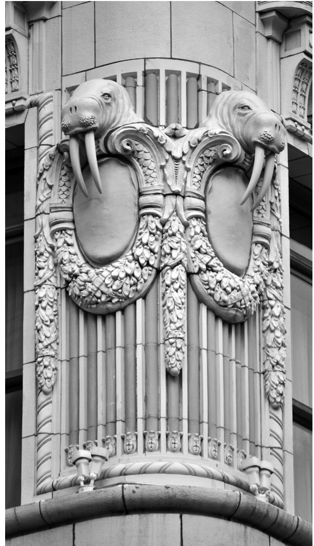
Fig. 1. The double walrus heads at the southwest corner of the Arctic Building in Seattle, Washington. Note the highly decorative terra cotta, bright colorful palette, and the tusks that hang from the walrus heads. (Credit: Brian Rich, 2013.)
