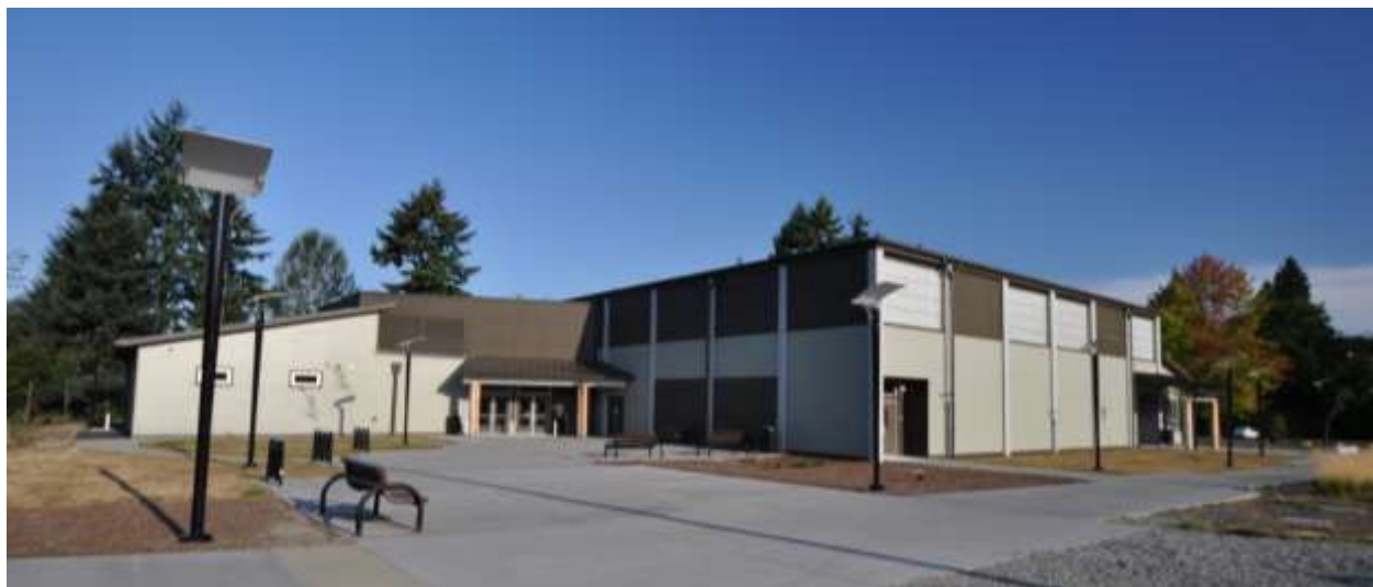
Figure 1: Exterior view of the gym at Lakota Middle School in Federal Way, WA. The existing concrete wall and wood framed roof structure of the 1950's gym was retained and renovated. The addition on the left is for locker rooms and ancillary spaces. Credit: Brian Rich, 2013.
