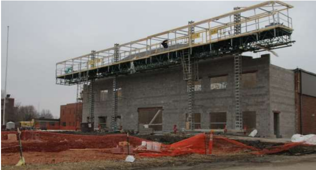
Figure 7: This gym is typical of the exterior CMU wall construction for Gym C. Note that the brick facing on the right edge of the photo is not included in Gym C.
