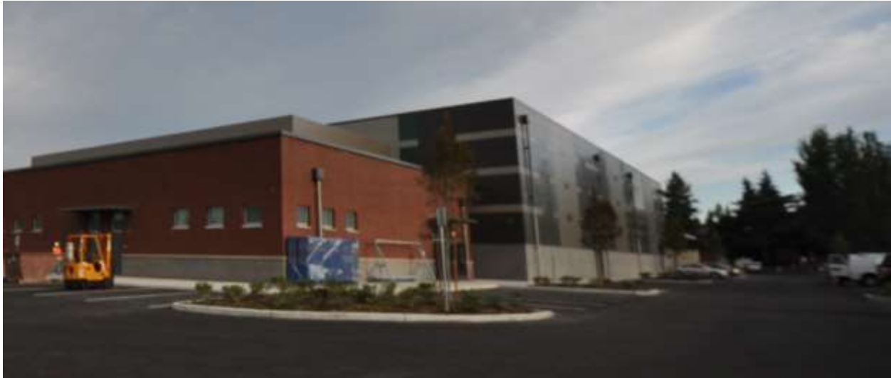
Figure 8: The Gym at Shorewood High school in Shoreline, WA is an example of Gym C construction. The main volume of the gym has CMU exterior walls and metal roof structure. The brick section at the left houses ancillary spaces not included in this LCA analysis.
