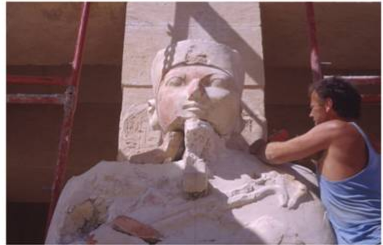
In-Kind Replacement with Dutchmen
