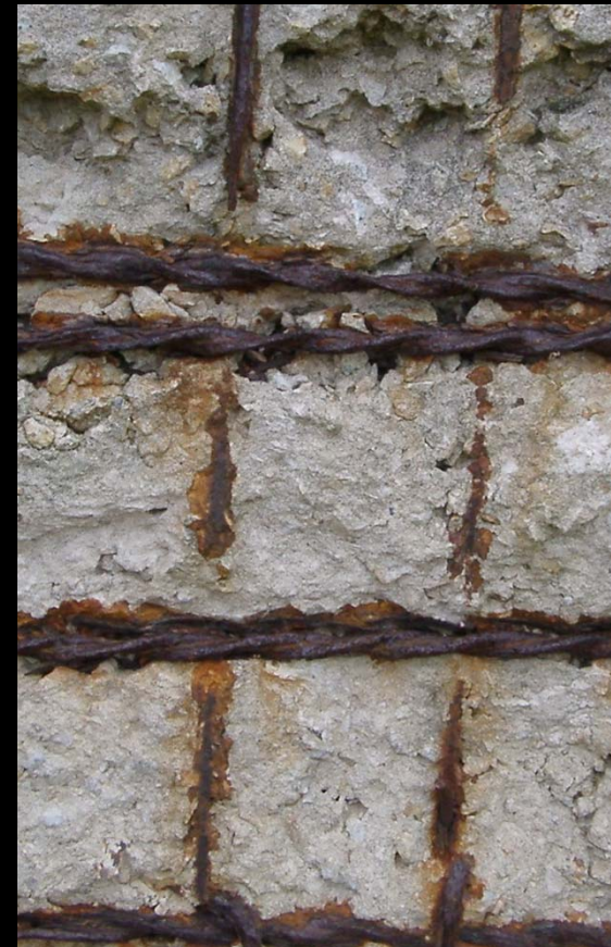
Figure __: Top left: Rebar placed too close to the surface of the concrete at the UW Seattle (credit: Brian Rich, 2014). Bottom left: A diagram of rebar deterioration due to water (credit: Pirro, 2012). Right: Deterioration of rebar placed too close to the surface (credit: ).
