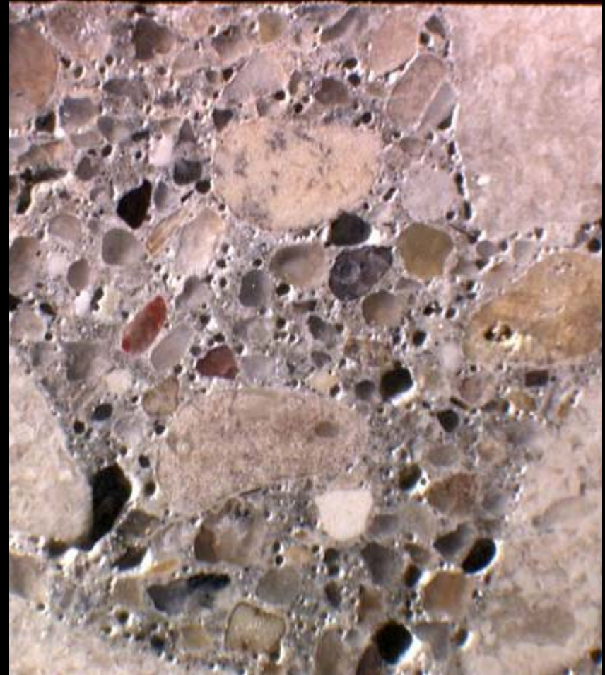
Figure __: Left: Exposed rebar corrodes and loses strength (credit: jenicke.com, 2012) Right: Air entrainment voids in concrete make space for water to expand into (credit: nist.gov, 2009)
