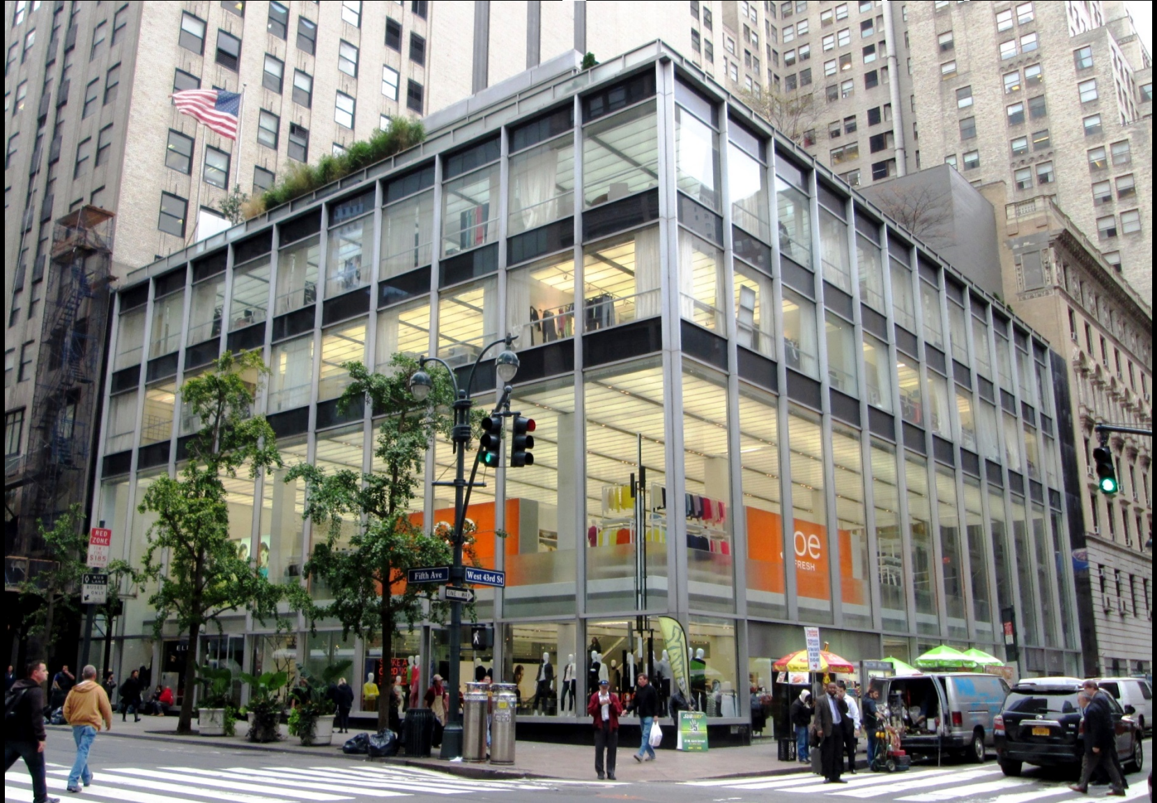
Figure __: The Manufacturers Trust Hanover Building in New York exemplifies the extension of the exterior envelope into the interior ceilings, floors, and walls. Credit: wikiwand.com
