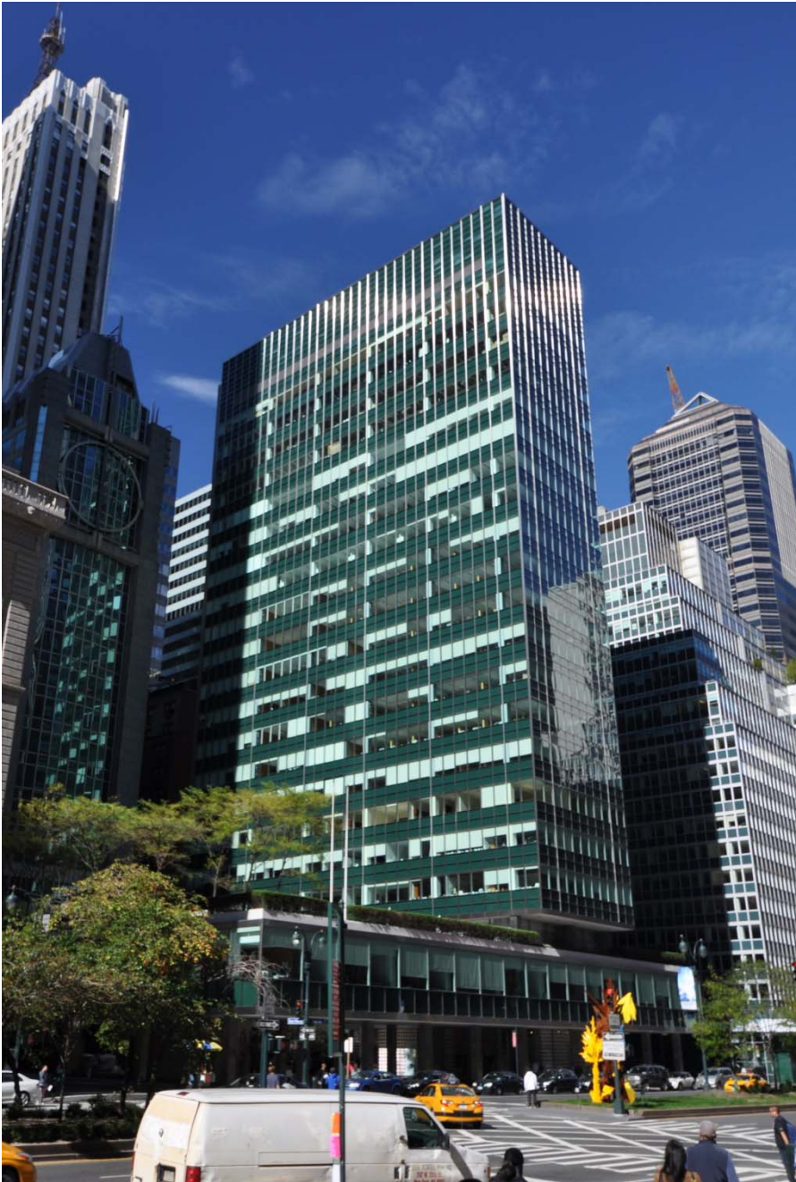
Figure __: The Lever House by Gordon Bunshaft of SOM is one of the earliest aluminum curtainwalls in New York. Credit: Brian Rich, 2013
