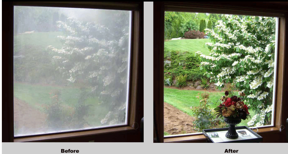
Figure __: The window on the left is an example of a failed insulated glass unit. Credit: lakelandglassmirror.com
