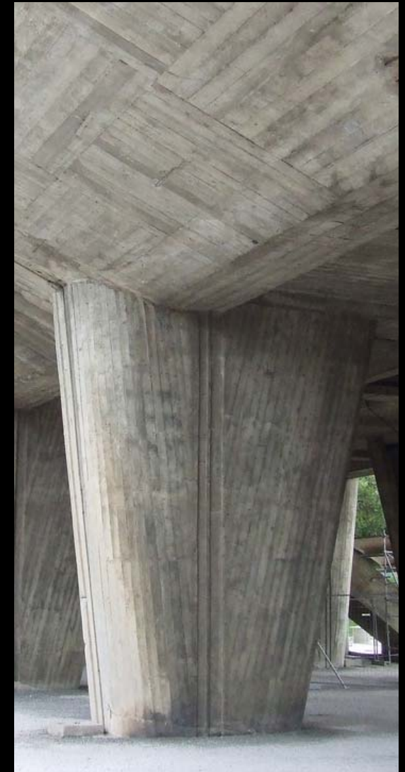
Figure __: Left: The main building at the Ballard Locks with exposed aggregate concrete, 1911-1917. (credit: Brian Rich, 2013) Right: Board formed concrete at the Unite D'habitation by LeCorbusier, 1952. (credit: Piere Janerete, 2014)
