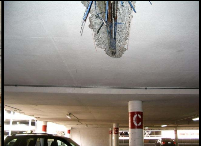
Figure __: Top: Components of a flat duct post-tensioning system (credit: ptsindia.net, 2015). Bottom left: Deteriorating tendons (credit: KJ Rodgers, 2013). Bottom right: Failure of post tensioned tendons can destroy the concrete cover as well (credit: cowleyengineering.com).
