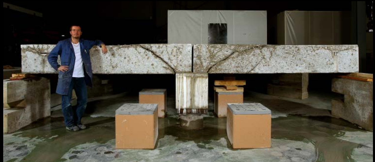
Figure __: Photos showing concrete “punching” on the bottom right (credit: http://ibeton.epfl.ch/recherche/punching ) and two methods for reinforced concrete to prevent punching shear at column to slab connections. The Duluth MN Armory at the left and a “drop cap” at the right.
