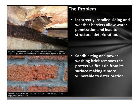
Again, interventions intended to repair and make the building viable and attractive for the long term future have caused irreversible damage to the building. Major repairs are necessary to mitigate the reduction of the service lives of these buildings. No matter how successful the mitigation, though, historic fabric has been lost and cannot be replaced.
