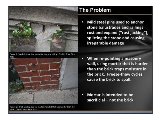
Too often mild steel is used for structural support and rusts when the building envelope no longer protects it. Proper maintenance, in some cases, would prevent subsequent rust-jacking and spalling. However, it is the original design that is at fault in the first place for not anticipating the problem.
